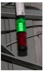
The sample areas are accessed through interlocked doors. The key to the locks must be inserted and turned in the trap box before the shutter can open. When the key is in and turned and the shutter requested out of the beam line, the green light above the beam line will turn red indicating that the shutter is out and beam on. The key at this time is trapped and cannot be removed.
